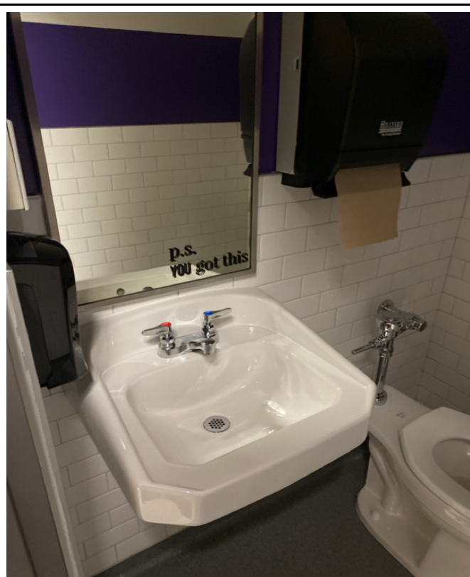
2/6/2024 - 327-26 - Elementary School - Room 38 - Right Restroom
