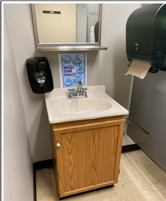
2/6/2024 - 327-1 - Elementary School - Dome - Girls Restroom
