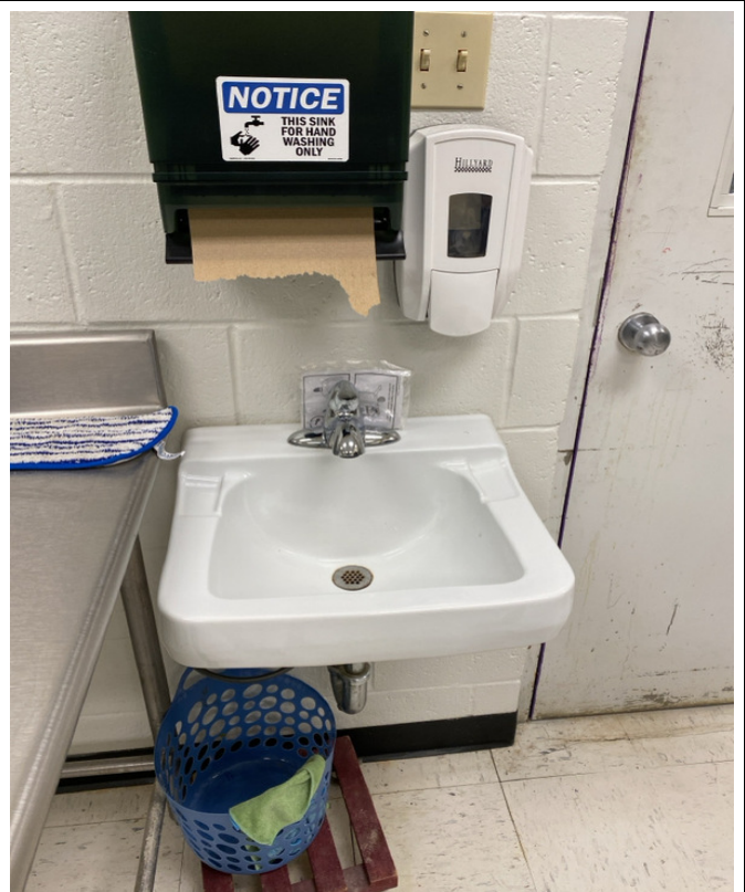
2/6/2024 - 327-6 - Elementary School - Kitchen - Handwashing Sink
