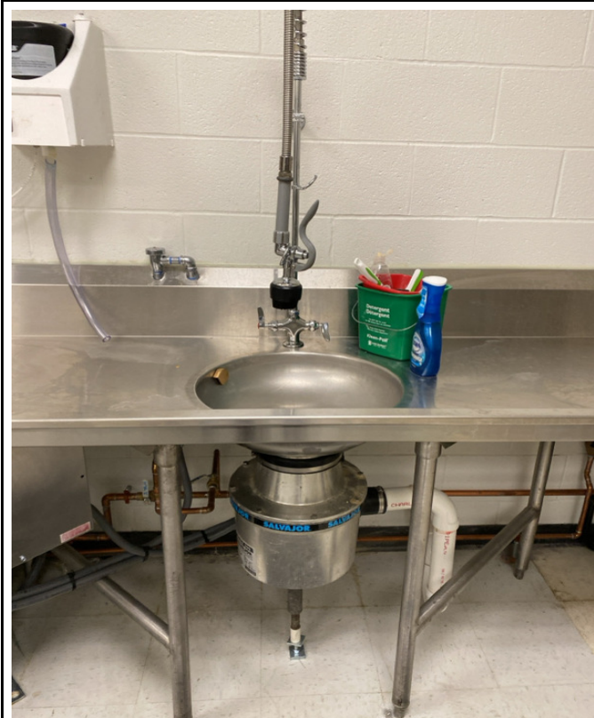
2/6/2024 - 327-7 - Elementary School - Kitchen - West Sink
